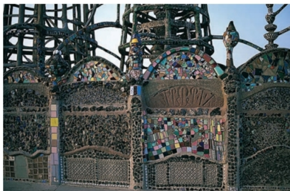
1.4 Sabatino “Simon” Rodia. Nuestro Pueblo . Top: distant view. Bottom: detail of enclosing wall with construction tool impressions. 1921–54. Mixed media. Height 100'. Watts, California.
